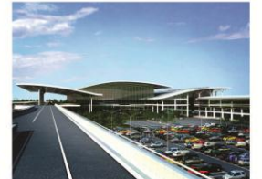
Noi Bai International Airport
